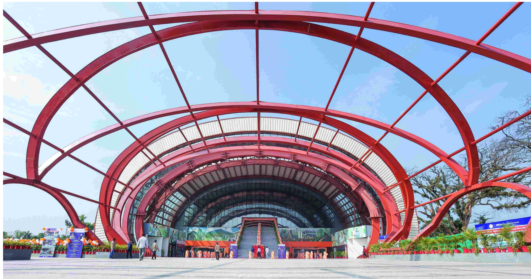
New Passenger Terminal Building Petrapole - West Bengal
